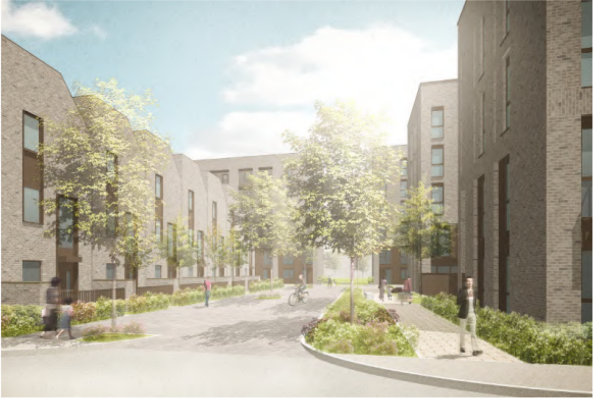
View along route to Newlands Park from Stebbing Way (between blocks C,D & E)
